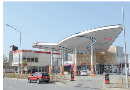
A Haengbok multi-purpose gas station in Incheon.
