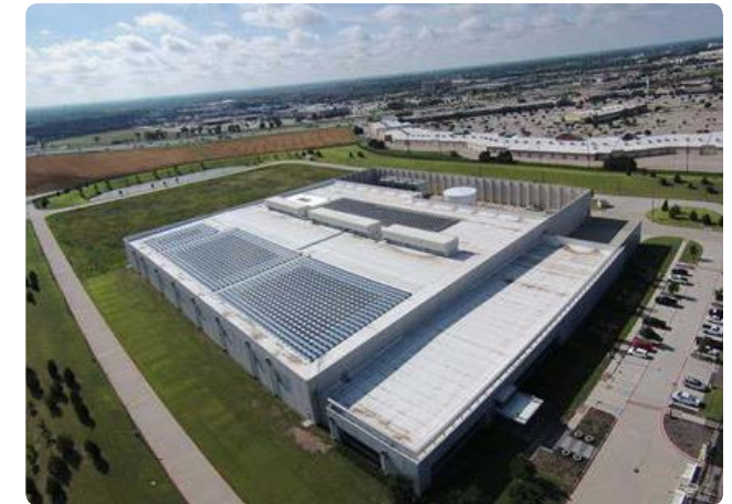
Cisco's Allen, Texas, Data Center Solar Project
