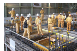
Finding multiple defects concealed in a model construction site
