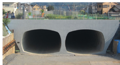
View of the tunnel entrance of the Kawajiri Tunnel at Sagami Longitudinal Expressway Project
