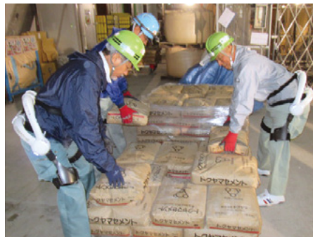
Skilled construction workers wearing HAL® lift a (25 kg) bag of cement
