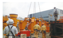
Assembling a tower crane platform
