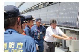
An Obayashi employee explains about the solar power facilities
