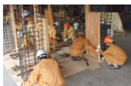
Assembling pillar reinforcement bars and concrete molds
