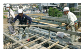
Assembling a scaffold
