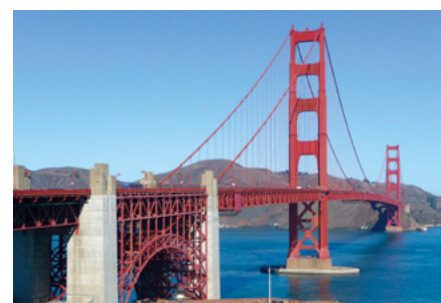
Golden Gate Bridge Seismic Retrofit (U.S.)
