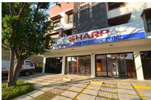
Exterior of the newly renovated Davao Branch Service Center
