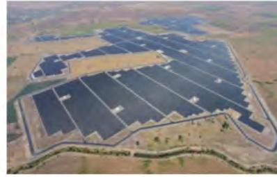
Mega-solar power plant in Thailand
