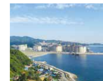
▼ 270,000 kℓ tank construction site at Samcheok Terminal Division
