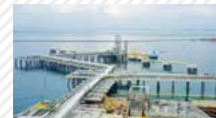
▼ PTT LNG Re-gasification Terminal Project, Thailand
