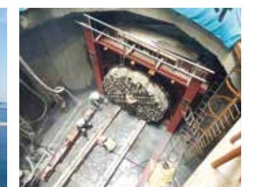
▼ Construction site for the main pipe semi-shield from Janglim to Jinhae
