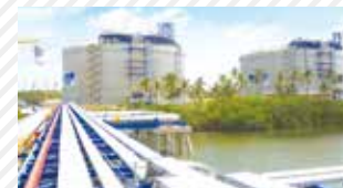
▼ Manzanillo LNG Re-gasification Terminal Project, Mexico
