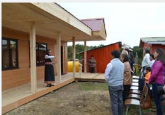
Construction of a preschool will allow children to learn and to gather in a common space.
