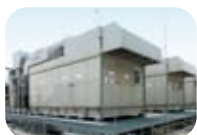
Private power generation equipment installation
