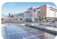
Solar panel installation
