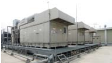
Private power generation equipment installation
