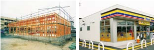
Store under construction MINISTOP store (FSC-JPN-0036 *FSC, A.C. All rights reserved.)
