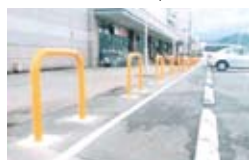
Parking Lot Guardrails
