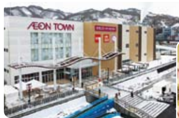
Aeon Town Kamaishi Opened in March 2014
