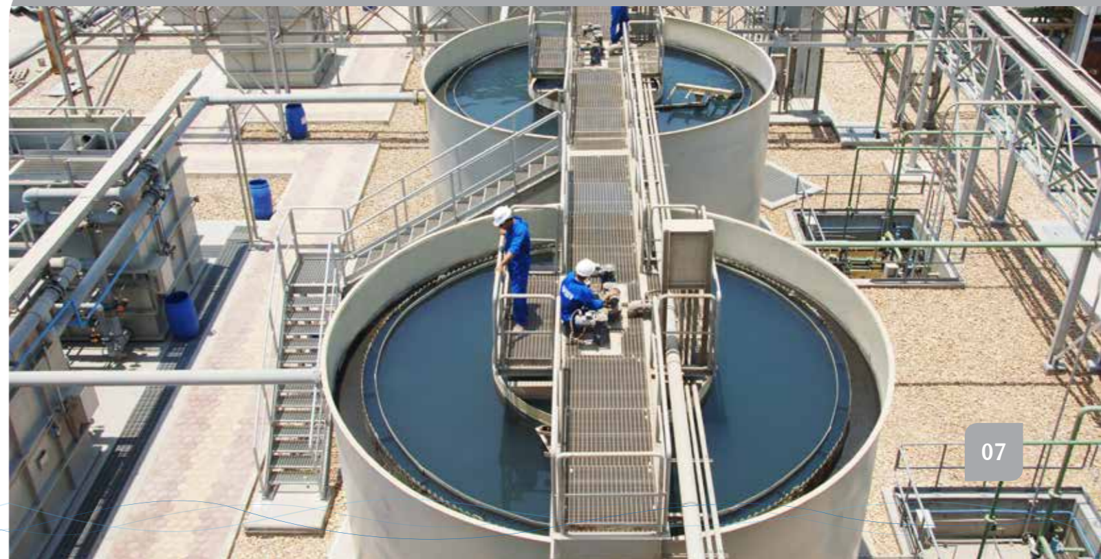
Metito Combined Cycle Project for El Kuriemat Power Station in Upper Egypt
