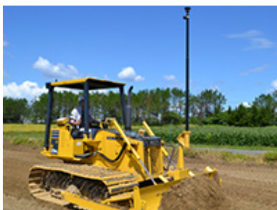
Leveling work by an intelligent machine control bulldozer
