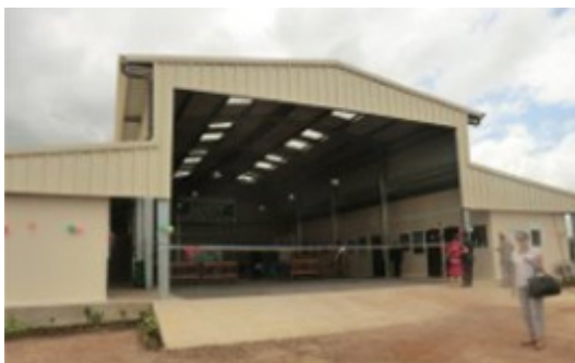
Japan Heavy Duty Equipment Operator School (SHDEOS), opened in Liberia in June 2014
