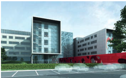
IMI Hydronic Engineering has installed its newest and most efficient balancing & control solution into the ALMA Hospital, Eelko in Belgium, which will help the customer to meet their efficiency targets.
