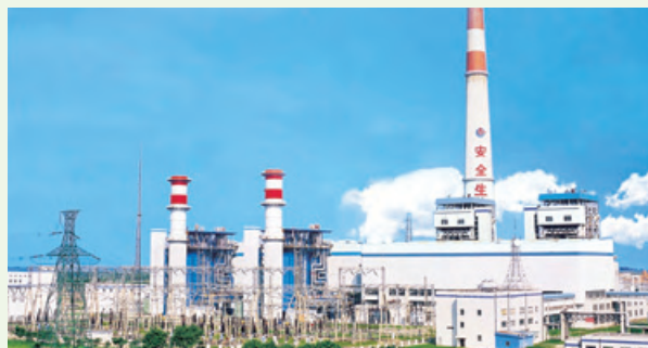
CNOOC Zhongshan Jiaming Power Plant
