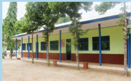
School buildings when handed over in November 2014
