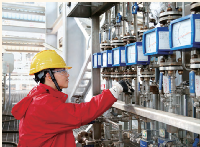
Equipment repair & maintenance for Huizhou Refinery
