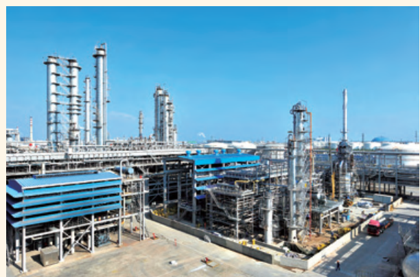
The full range FCC gasoline hydrodesulfurization unit of Huizhou Refinery was put into production.
