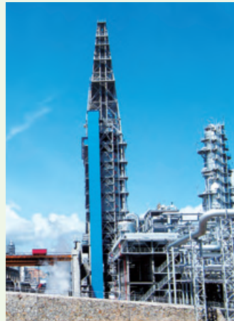
Factory Area of Huizhou Refinery
