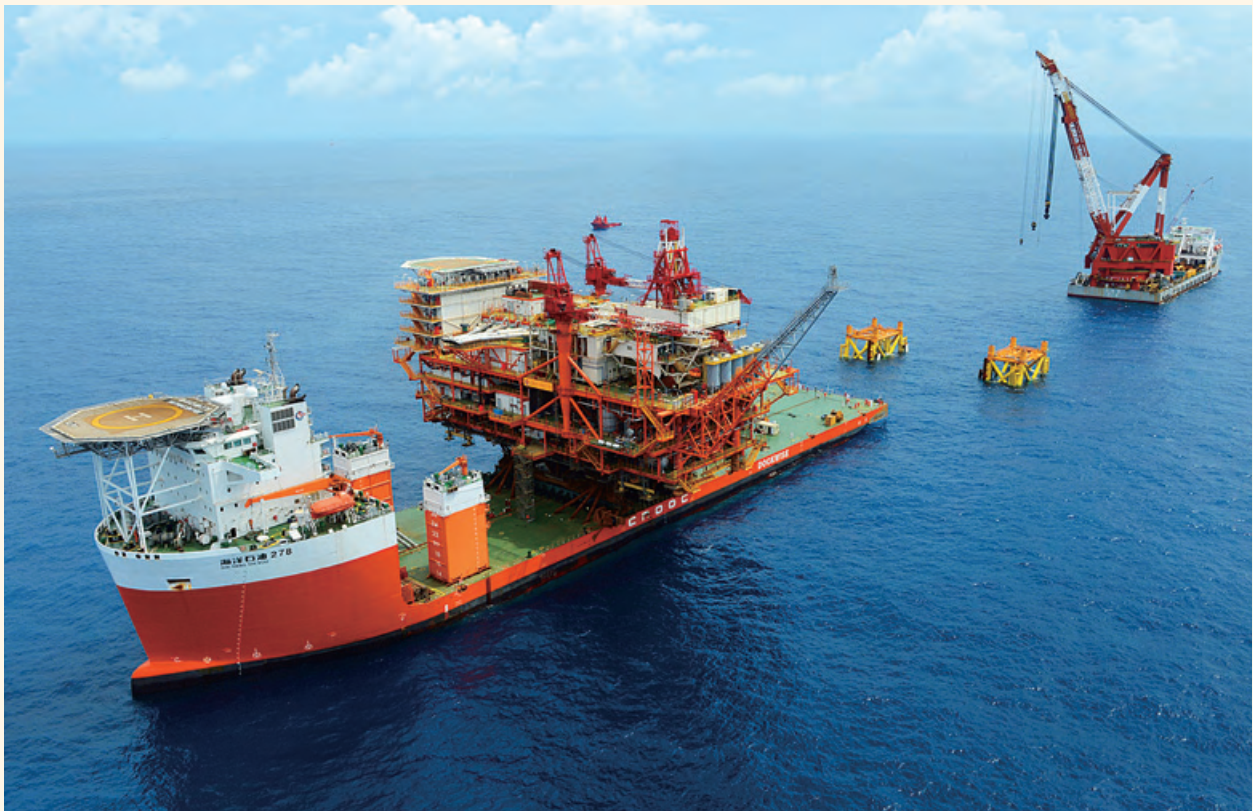
“Float-over” installation of offshore platform is ongoing.
