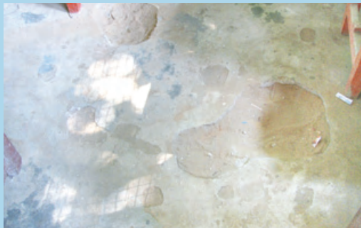
School buildings before reconstruction and decoration
