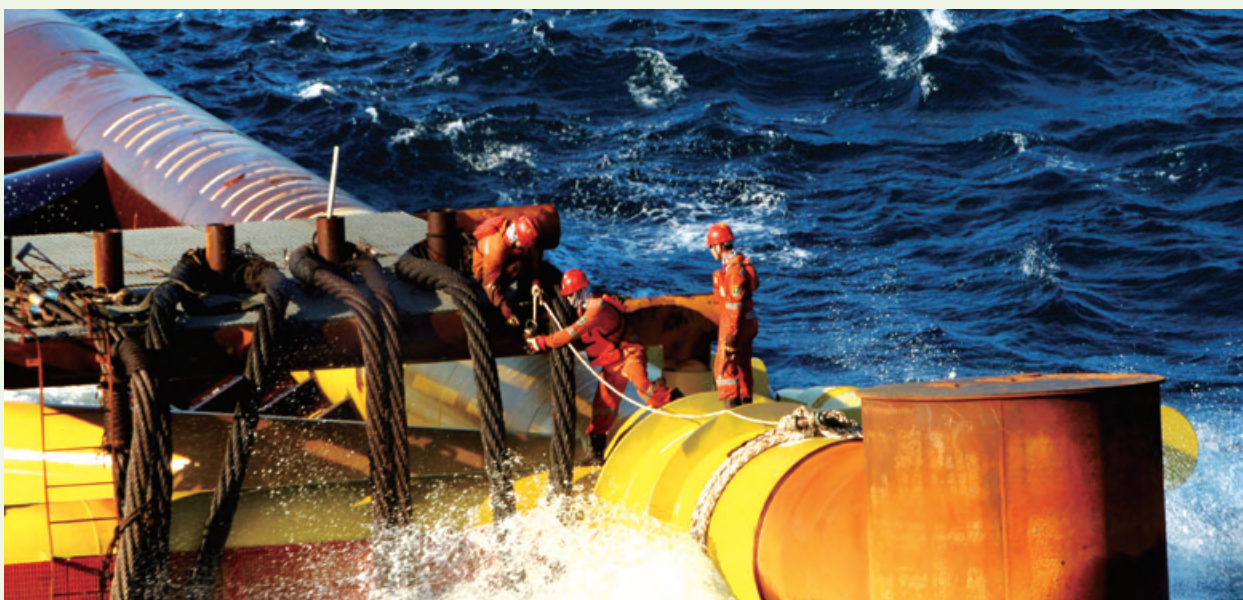
Lishui 36-1 Project is under construction.
