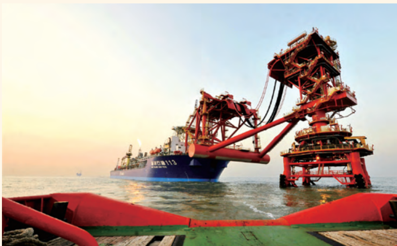
FPSO of Bozhong 25-1 Oilfield
