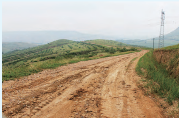
Before and after the highway open to traffic
