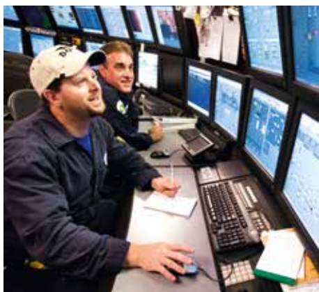
▲ Technicians monitoring activity in the control room of the Atlantis platform in the Gulf of Mexico in the US.
