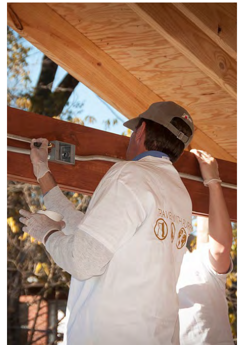
Hilton Worldwide Team Members work on construction projects during Global Week of Service, November 2012.
