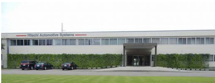
Gunma Works, Hitachi Automotive Systems, Ltd.
