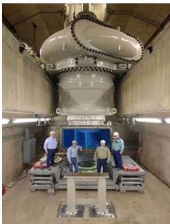
Four-stage turbine pump
