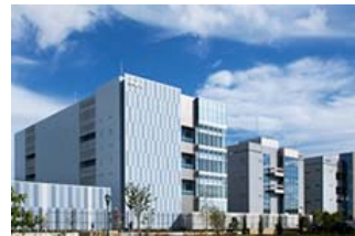
Data Center (Okayama No. 3 Center)
