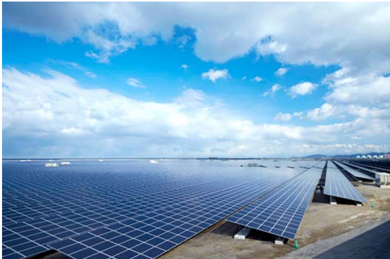
This mega solar power plant on a 105-hectare site in Oita City, Oita Prefecture, has around 340,000 solar panels and a capacity of 82,020 kW. It is forecast to generate 87 million kWh per year (the equivalent annual power consumption of around 30,000 households). *1
