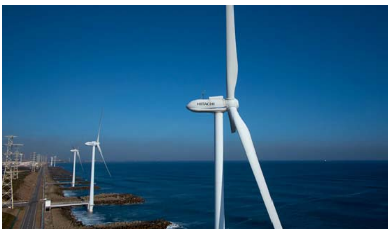
Wind Power Ibaraki Co., Ltd., Kamisu Wind Farm The Kamisu Wind Farm, where turbines are fixed to the seafloor, is offshore of Kamisu City in Ibaraki Prefecture. The 15 downwind turbines making up Hitachi's 2000 kW wind turbine generation system have a total output of 30,000 kW.
