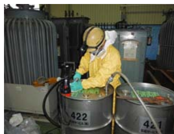
Removing oil from electrical equipment contaminated with low PCB concentrations
