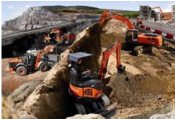
Heavy Plant Training Centre
