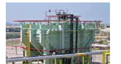
Commercialization of LNG carrier cargo tanks
