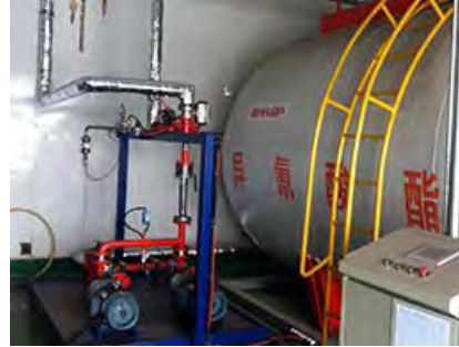
(After) Transporting isocyanate using tanks
