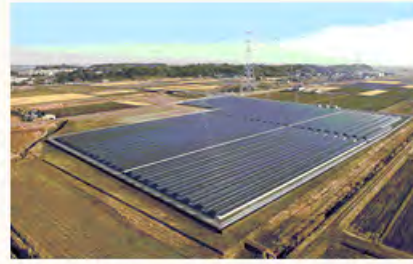
Tonemachi Sharp Solar Power Plant (Kita-soma District, Ibaraki Prefecture, Japan)
