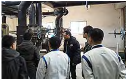
On-site inspection to renew Cleaner Production certification
