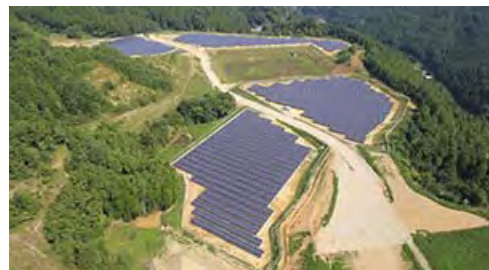
Sharp Miyoshino Solar Power Plant (Yoshino District, Nara Prefecture)
