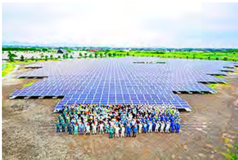
Sharp solar modules and construction workers
