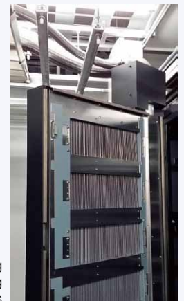
Cooling equipment using phase change cooling technologies
