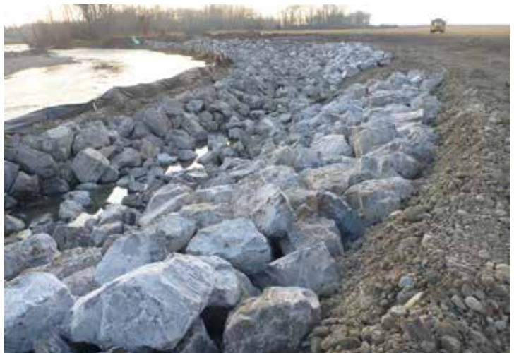
New riverbank protection measures under construction
