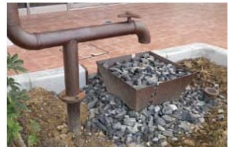
The Rain Garden™ project to filter rain water through top soil instead of transmitting it directly to sewage pipes
