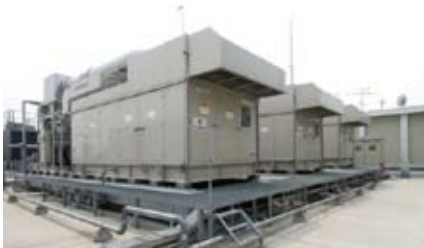
Private power generation equipment installation
