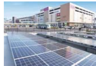
Solar panel installation
