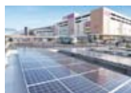
Solar panel installation
