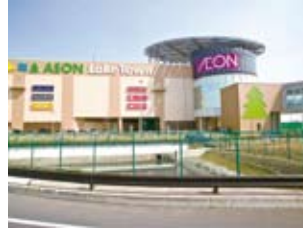
Aeon Laketown Our 8th Eco Store, installed solar panels to be domestic commercial facility's largest.
