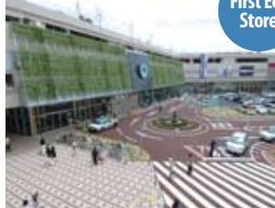
Aeon Town Chikusa Introducing a solar power and wind power
