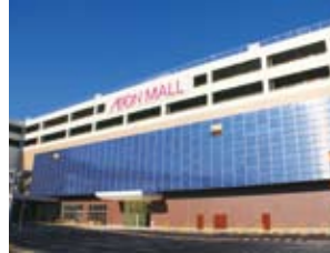
Aeon Mall Funabashi Our 12th Eco Store, turned into an LED 97.6% of the lighting of the entire facility.
