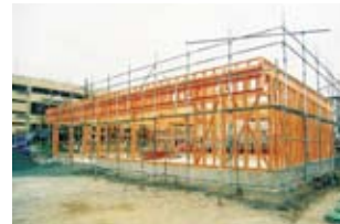
Store under construction
