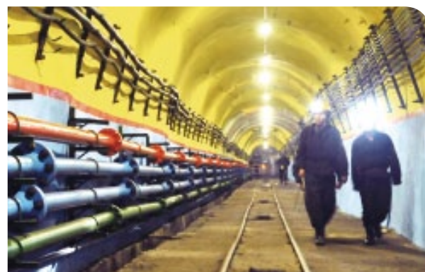
Passageway in the mine of Huating Coal Industry Co., Ltd
