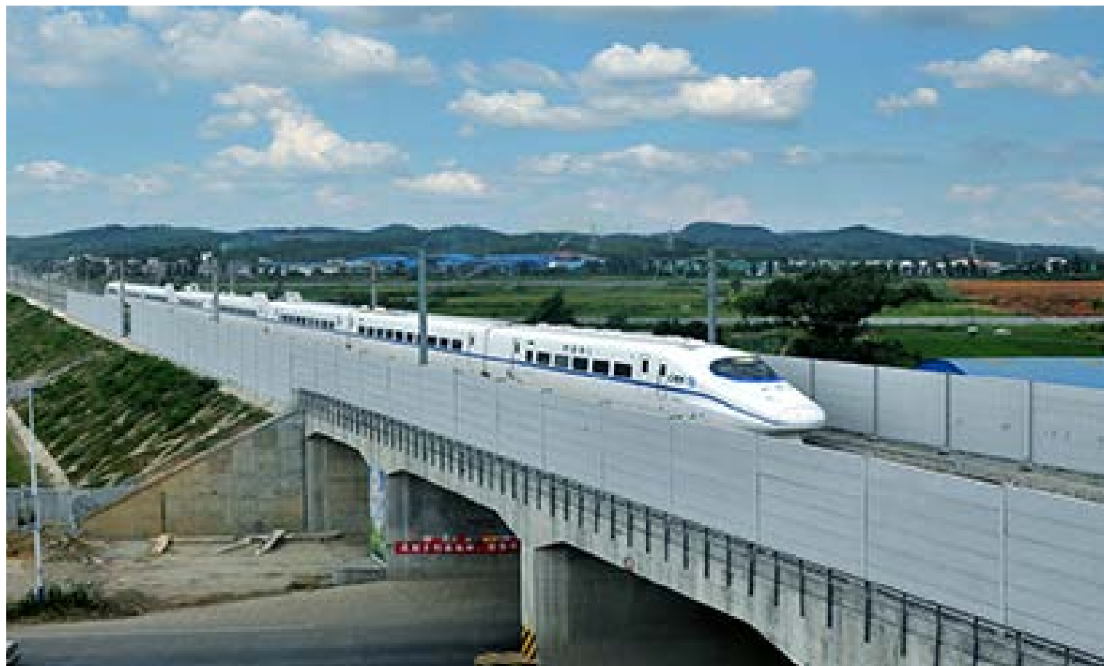
广西高铁线路 A high-speed railway in Guangxi
