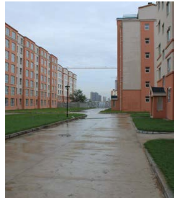
改造后 After Transformation
