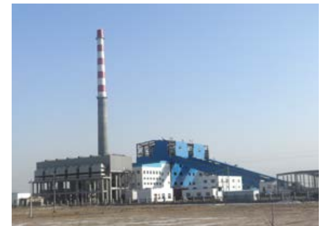
寿阳生物质发电项目 Bio-power plant in Shouyang County
