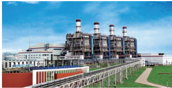
CNOOC Gas & Power Group's gas power plant in Putian, Fujian
