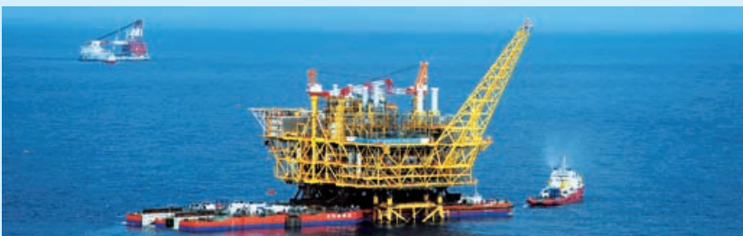
(4) Butt jointing between platform and jacket when tide is out
