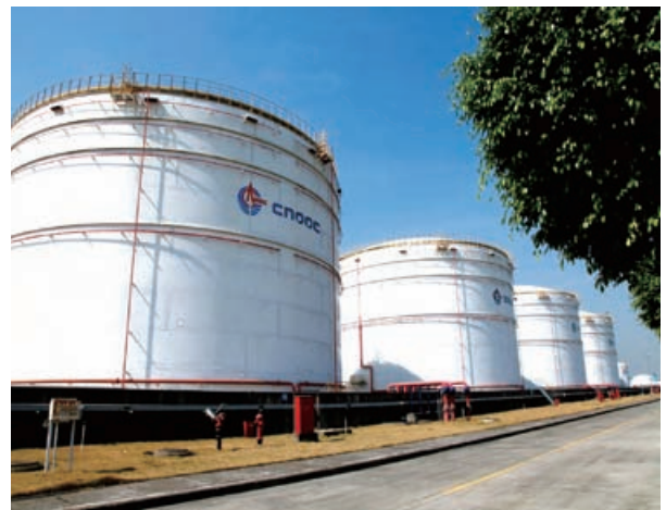
Dongguan Lisha Oil Storage Tank
