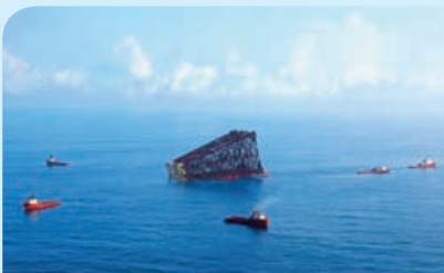
(1) Installing jacket
