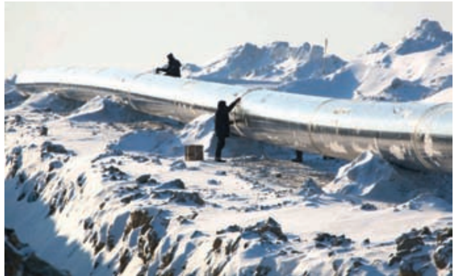
↑ Pipeline inspection in the Russian Arctic.
