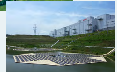
Floating 200 kW solar power generation system set up in cooperation with Kameyama City on a stormwater retention pond that is adjacent to the factory. Proof-of-concept tests are underway.
