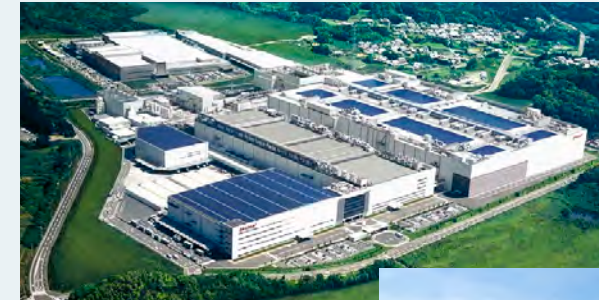
5,210 kW solar power generation system installed on the roof and walls at the plant
