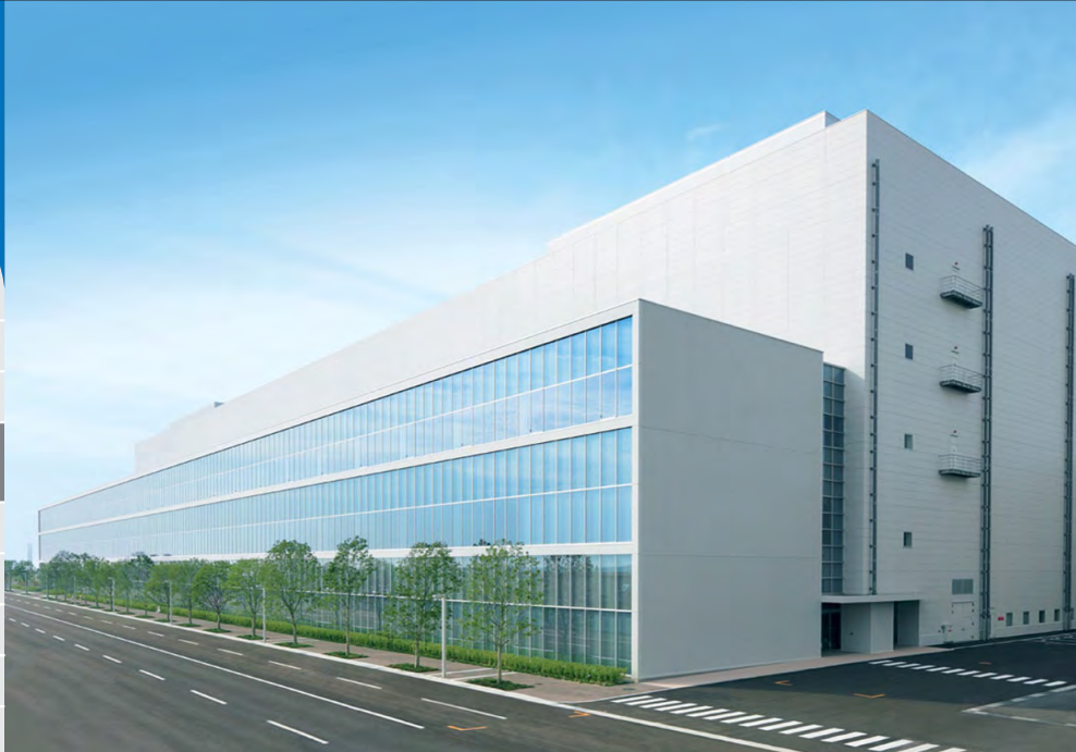
Solar cell plant at GREEN FRONT SAKAI that began operations in March 2010
