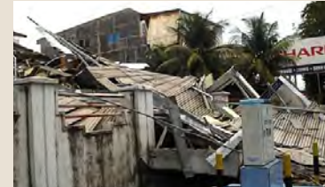
The SEID branch in Padang was damaged in the Sumatra earthquake
