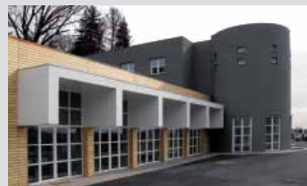
A new "We Parents Onlus" day centre at Erba (Como) for the care and physical and mental rehabilitation of the disabled.
