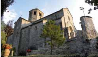
Restoration of the San Salvatore Monastery at Capo di Ponte
