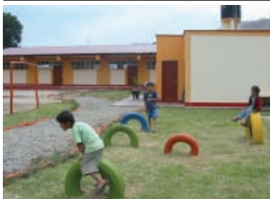
▼ School Rebuilding in Peru ▼
