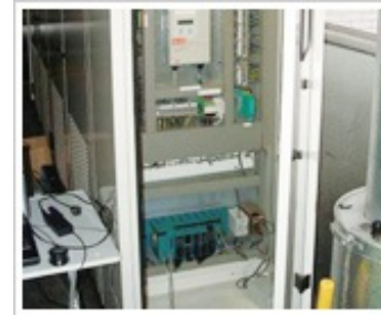
STARDOM controller installed in the site cabinet
