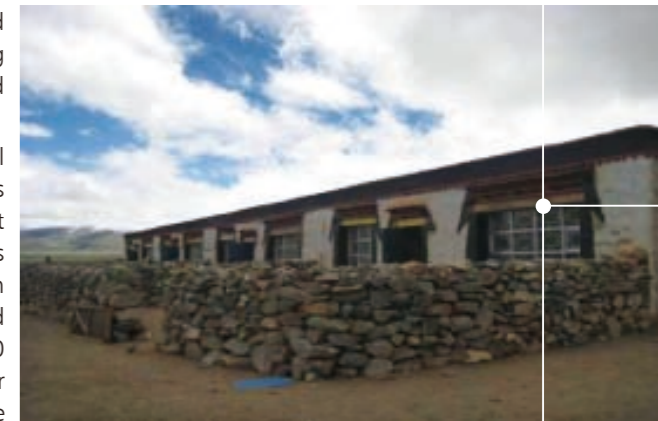
Assistance for Settlement Construction for Herders in Nima County of Tibet
