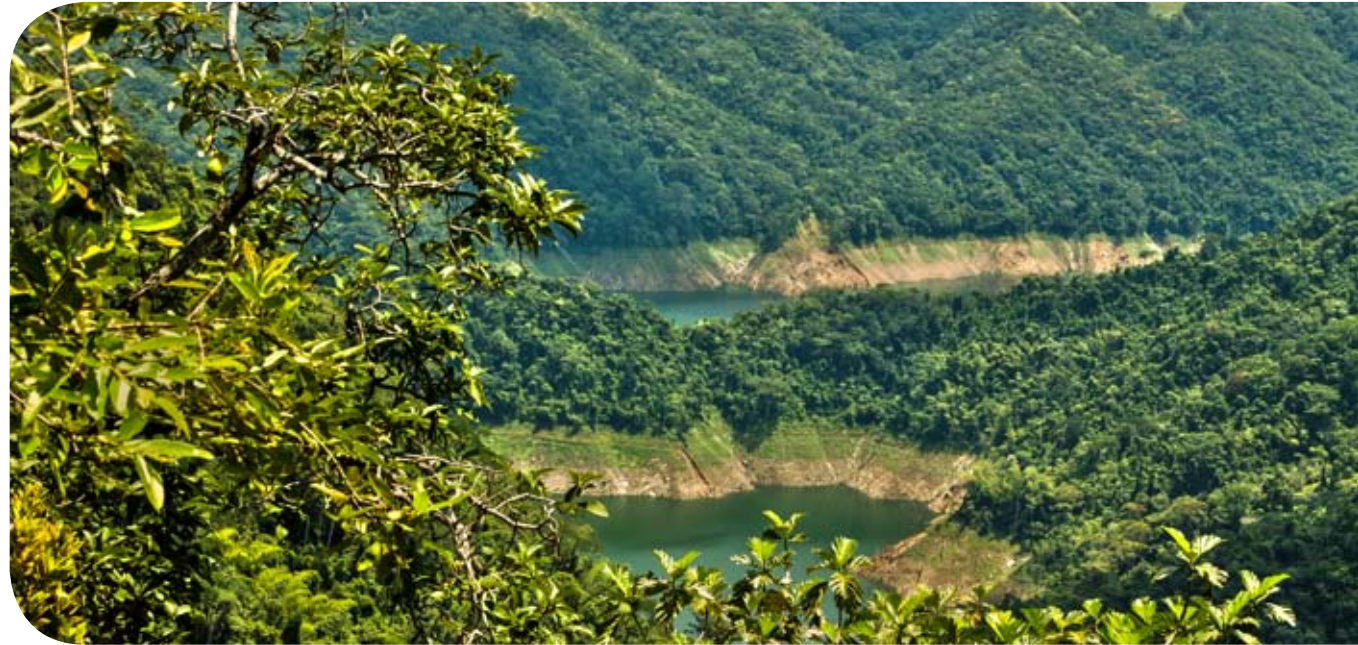
Amani Reservoir, Miel I Power Plant
