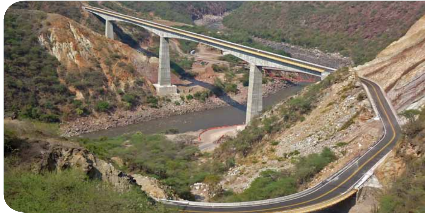
Guillermo Gómez Ortiz Bridge
