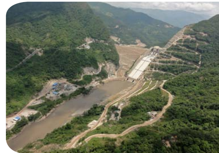
90% progress in the Sogamoso Hydroelectric Power Plant.
