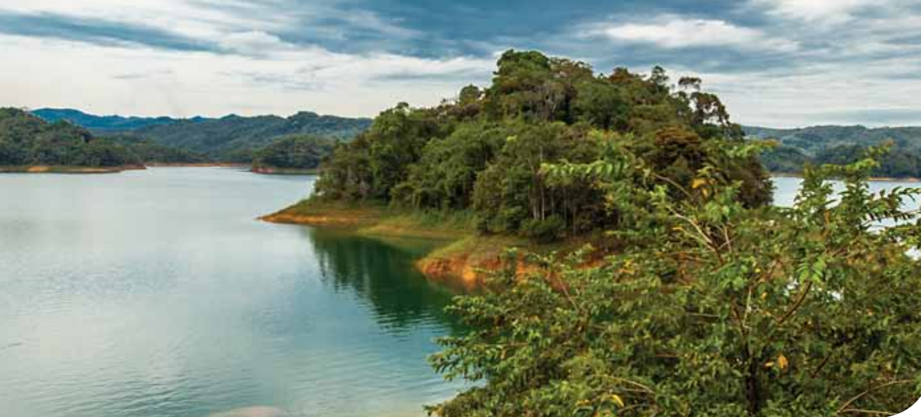
San Lorenzo Reservoir, Jaguas Power Plant
