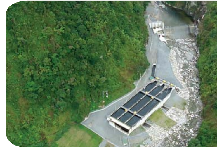
Inauguration of the Amoyá River, La Esperanza Hydroelectric Power Plant
