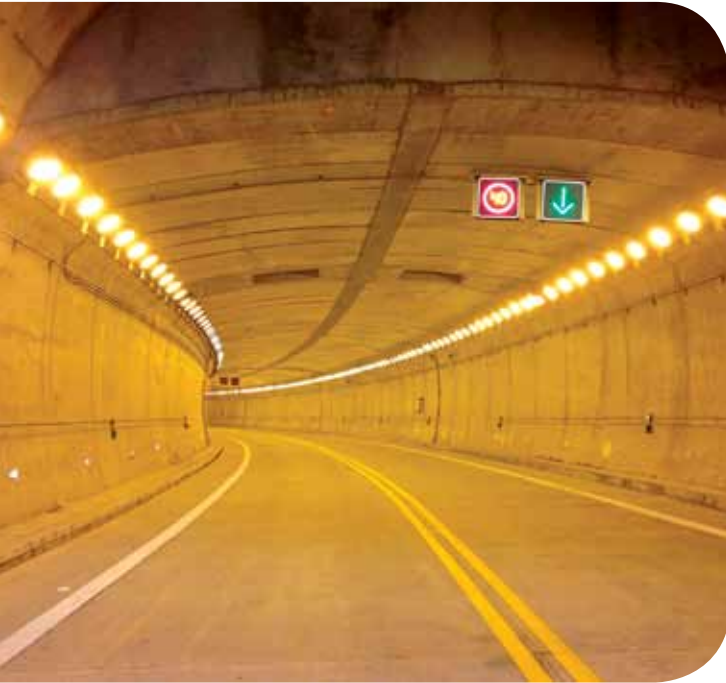
Road Tunnel I
