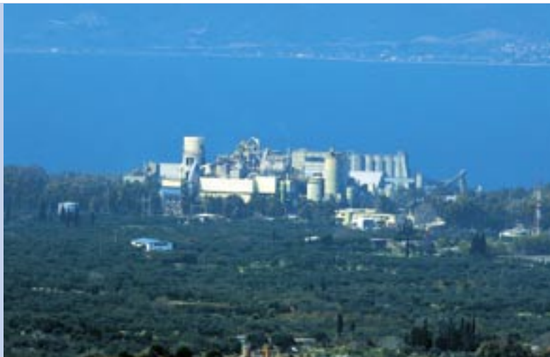
Patras plant, Achaia-Greece
