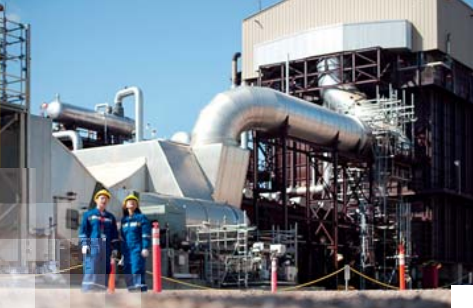
Our Quest CCS facility being built at the Scotford Upgrader in Alberta, Canada.
