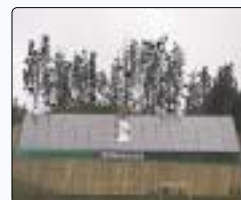
▶120kW photovoltaic generation
