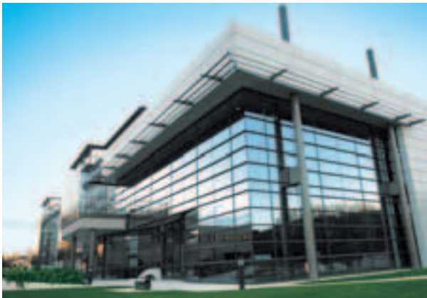
▲ In Vélizy (France), installations in new buildings enable a 40% energy saving.
