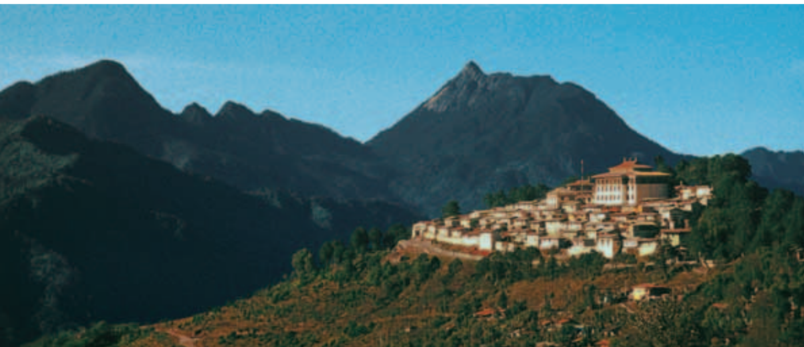
ALCATEL HELPS BRIDGE THE DIGITAL DIVIDE IN THE HIMALAYAS.
