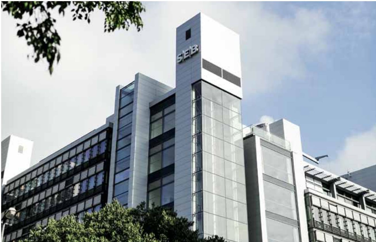
SEB's new headquarter in Frankfurt, Skylight, is optimised from an environmental and sustainable perspective, e.g. including LED lighting and detection sensors as well as recycled and low emission construction materials. The building will be minimum Leed Gold certified. Leed stands for Leadership in Energy and Environmental Design.
