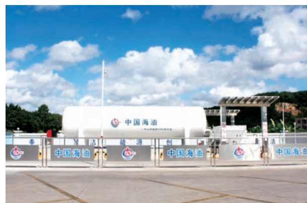
Zhongshan Chengnan Qiaozhuang Gas Station
