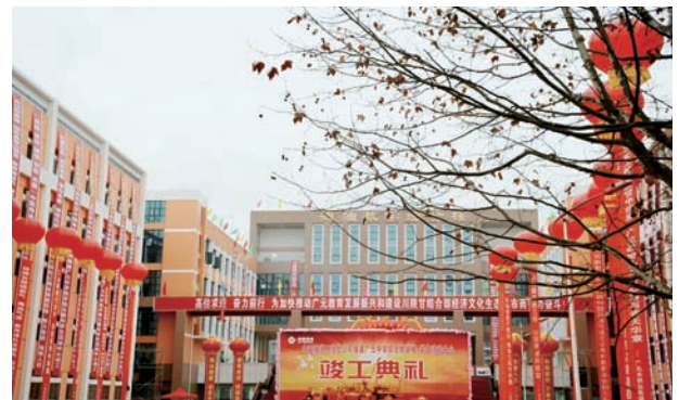
Construction of the CNOOC-financed multi-purpose classroom building at Guangyuan Middle School completed
