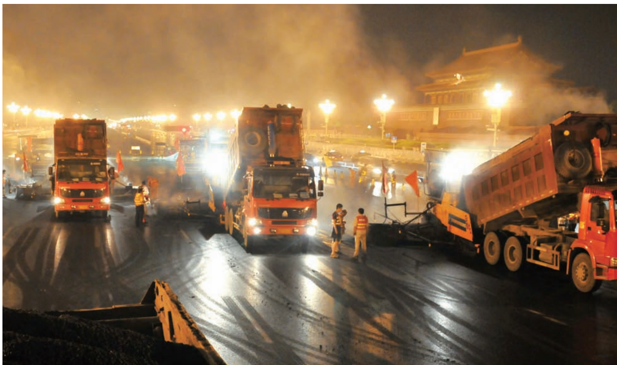
CNOOC 36-1 asphalt paves Chang'an Avenue
