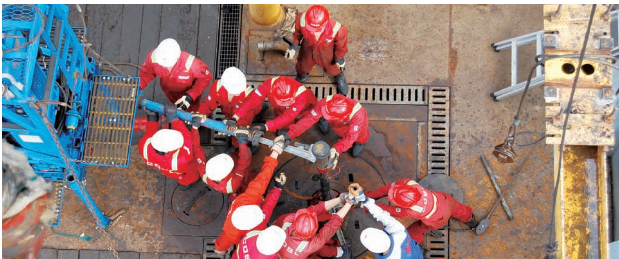
Well workover operation on an offshore platform
