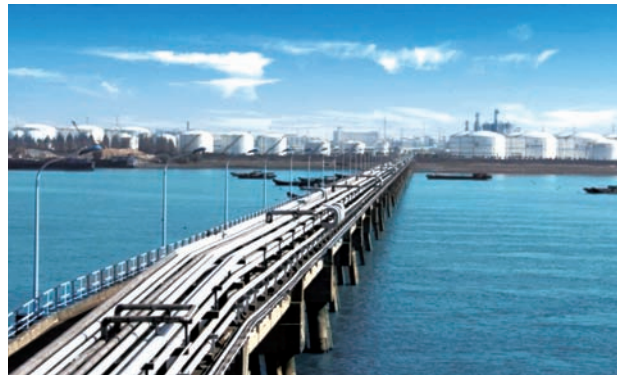
Nantong Huasheng Oil Storage Warehouses
