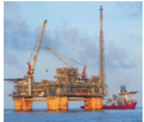
▲ The Na Kika platform in the Gulf of Mexico acts as a hub, gathering oil and gas from deep under the sea using over 100 miles of subsea pipes.
