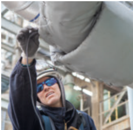
▲ A BP contractor measures the thickness of pipes at the Cherry Point refinery in the US.
