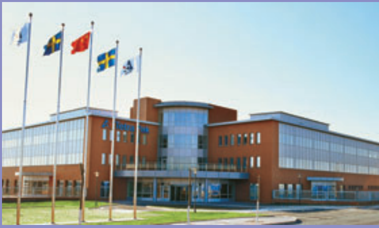
The new converting plant in Beijing demonstrates Tetra Pak's long-term commitment to growing in China.
