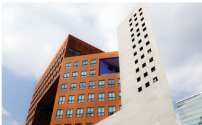
The recently opened corporate office building for Coca-Cola FEMSA in Mexico City meets the LEED Platinum certification in Core & Shell category.
