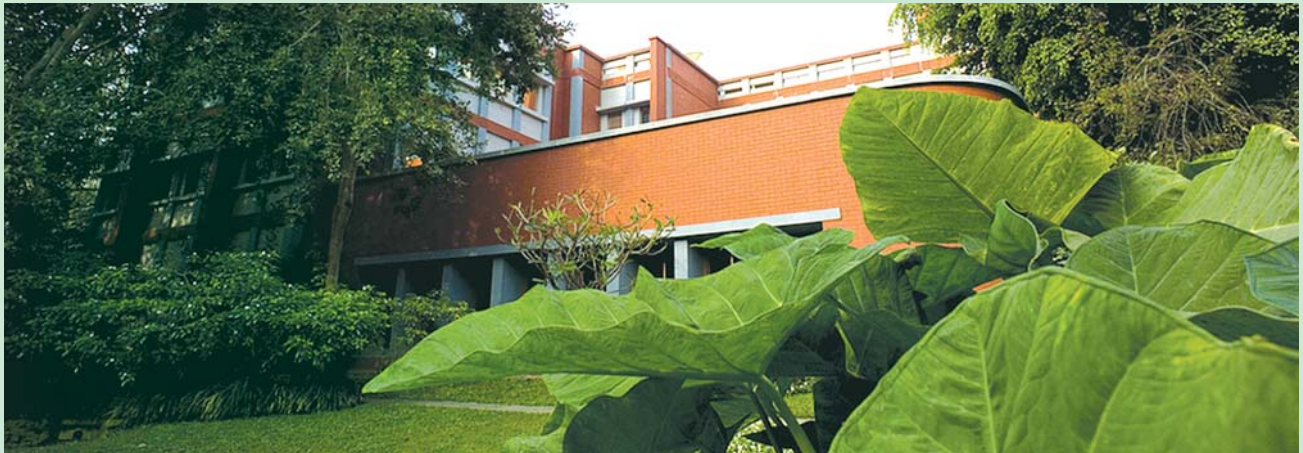
Green cover at the Bangalore development center, India
