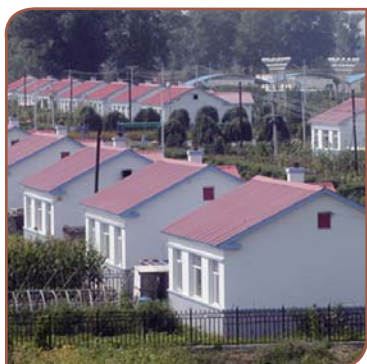
泥草房改造后 After renovation
