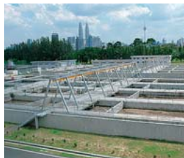
Bonus sewage treatment plant in Malaysia
