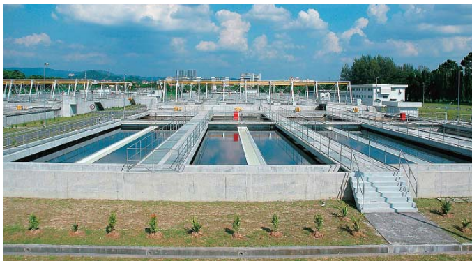
Bunus sewage treatment plant in Malaysia
