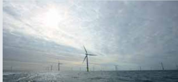
With 48 wind turbines and a transformer station out at sea, the Lillgrund offshore wind farm is one of the largest of its kind anywhere in the world.
