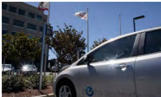
Electric vehicle charging at Cisco (San Jose, California)
