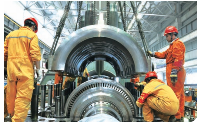
Equipment Installation and Debugging
