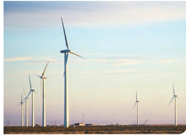
Huaneng Tongliao Baolongshan Wind Farm
