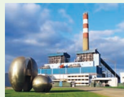
The first imported 600 MW supercritical coal-fired generating unit
