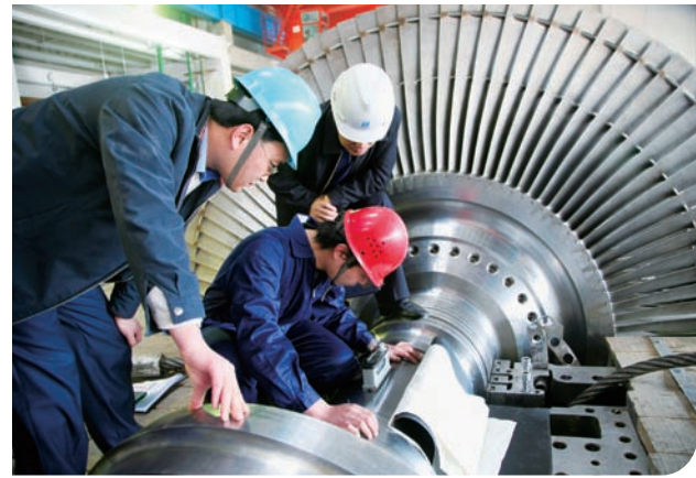
Equipment Inspection and Rectification
