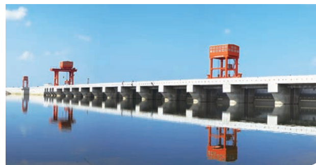
Huaneng Gezhen Hydropower Plant
