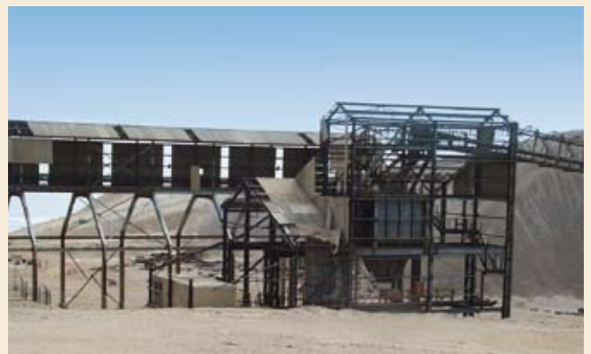
2. Any infrastructure not required for future use is removed
