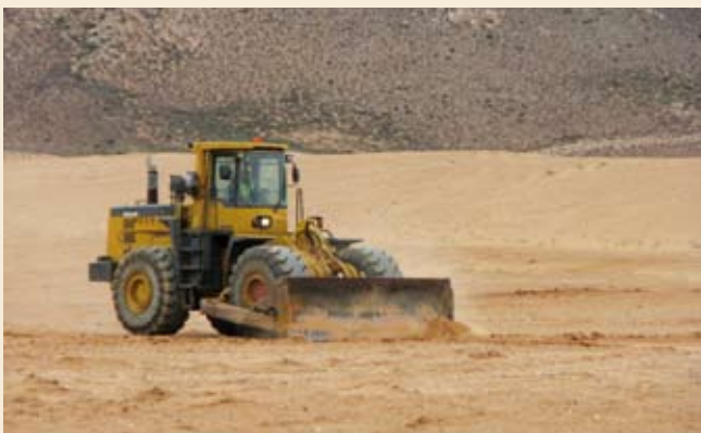
3. Where necessary, existing landforms are reshaped to their original structures. Current planning estimates that this will be required in 24% of the disturbed area
