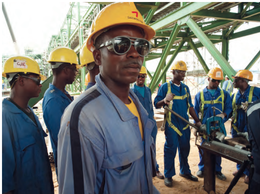
↑ Workers at the Gbaran-Ubie construction site.
