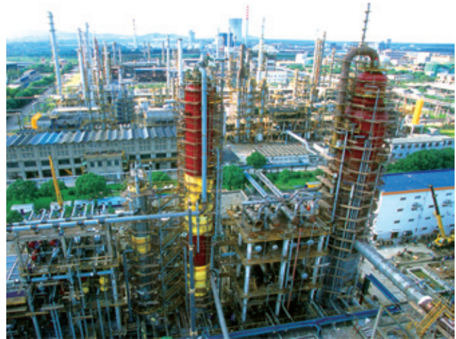
Zhenhai Refining & Chemical revamping construction site
