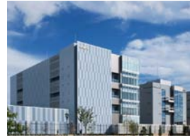
Data center (Okayama No. 3 Center)*
