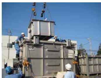
Loading PCB Waste for Disposal
