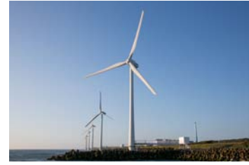
Wind Power Ibaraki Co., Ltd.'s Wind Power Kamisu 1 Offshore Wind Farm
