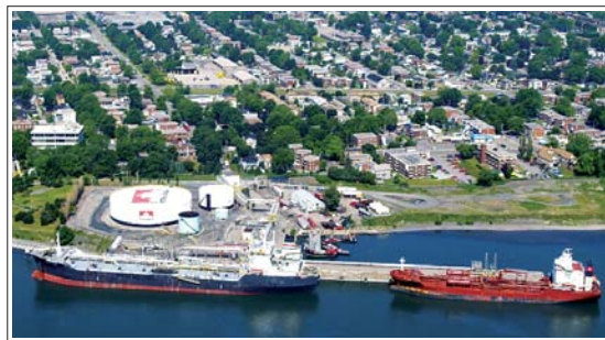
An aerial shot of Petro-Canada's Montreal dock.
