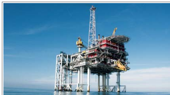
The only Petro-Canada operated offshore platform in Northwest Europe is the Hanze platform in the Netherlands sector of the North Sea. The F2-A-Hanze platform has been categorized by the Dutch authorities as "best in class" in terms of energy efficiency. In 2005, Hanze emitted less CO 2 than its permitted allocation. For both our Hanze platform and our new development (De Ruyter), energy efficiency plans are in place. For example, both platforms have waste heat recovery units and turbines with the best available technology for energy efficiency.
