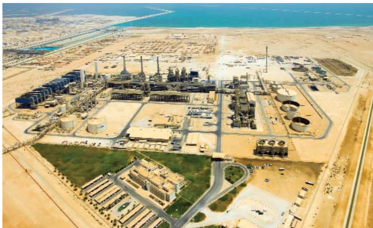
Oryx GTL in Qatar achieved a significant improvement in performance, production ramp-up and profitability
